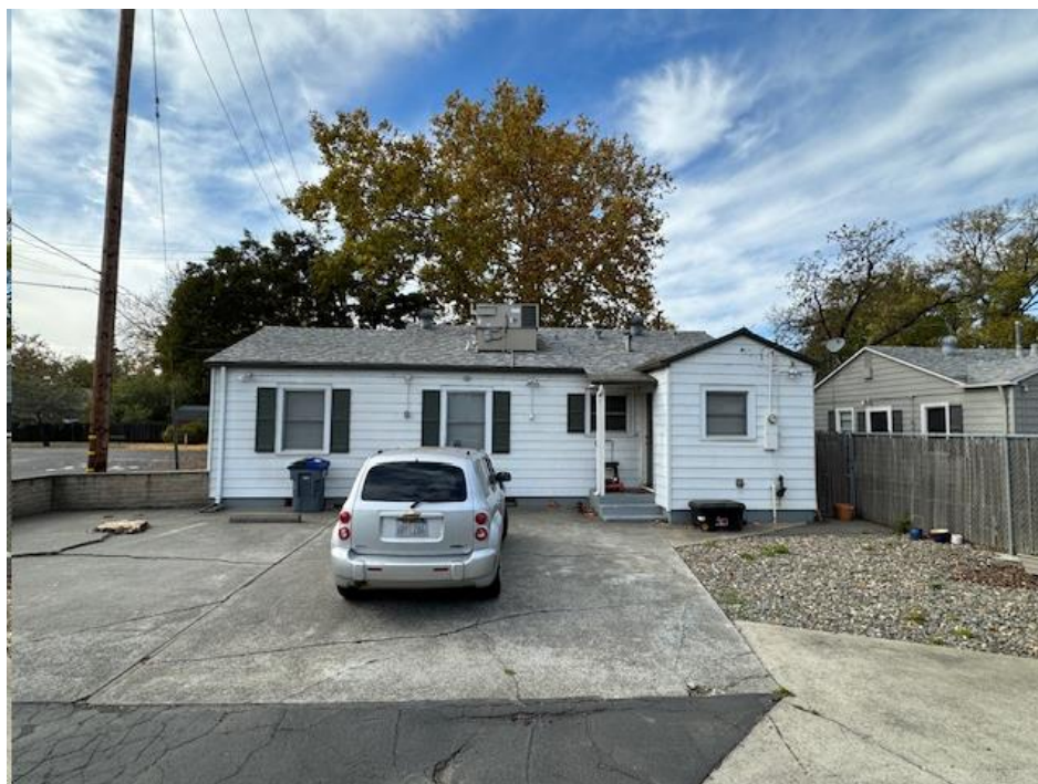
Photograph 4: View looking west at 724 G Street.
