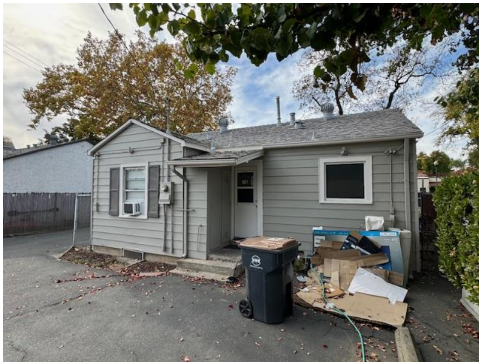
Photograph 4: View looking west at 730 G Street.
