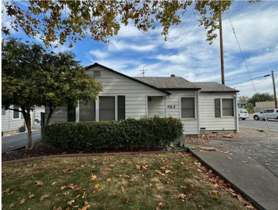
Photograph 1: View looking east at 724 G Street.
