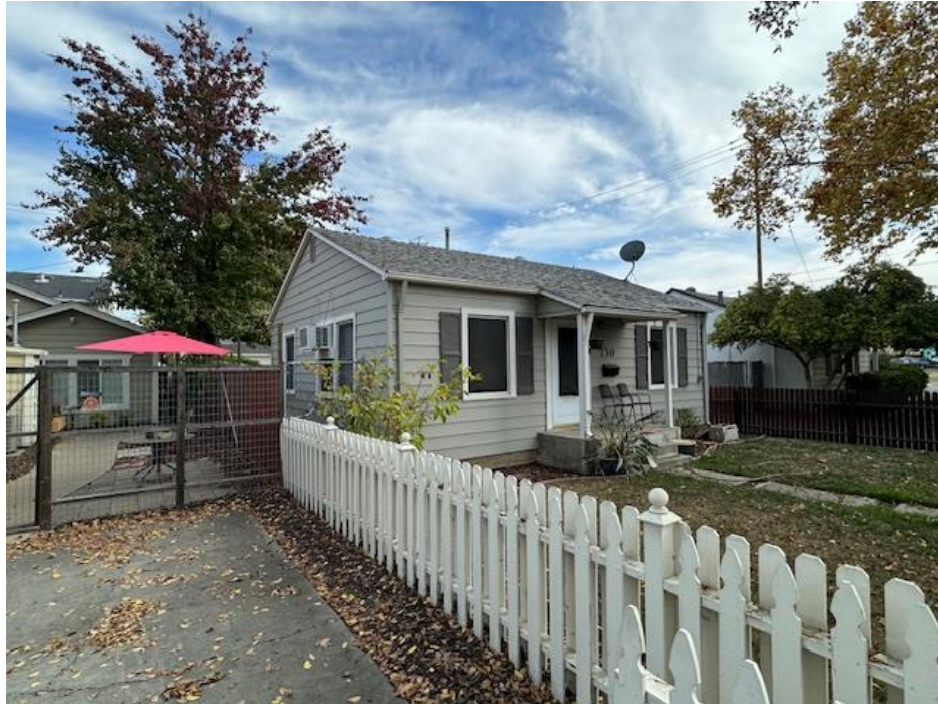
Photograph 1: View looking southeast at 730 G Street.
