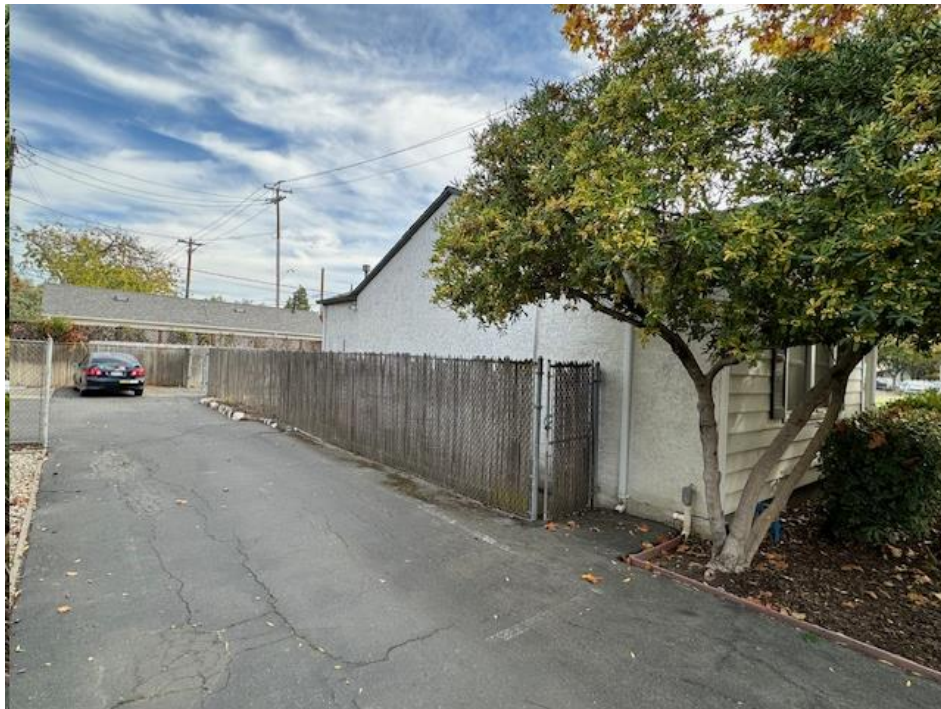
Photograph 6: View looking southeast at the north elevation of 724 G Street. Note the later application of stucco on this elevation.
